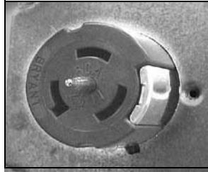
NEMA L6-50R wall receptacle (North America/Japan)
