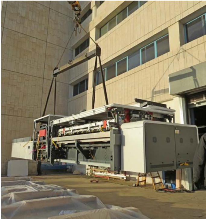
Figure 5-19 Lifting the Machine from the Pallet
