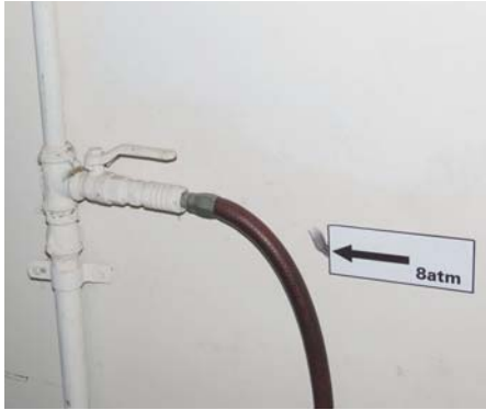
Figure 4-11 Compressed Air Connection to FB10000
