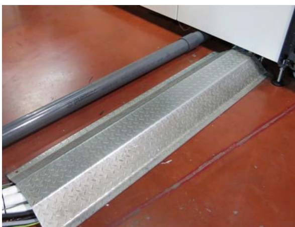
Figure 4-2 Covering the Inlet Pipes and Cables
