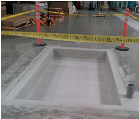
Figure 4-20 Pit for Unloader Lift
