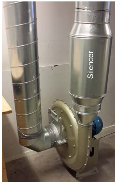
Figure 4-17 UV Extraction Fan Silencer
