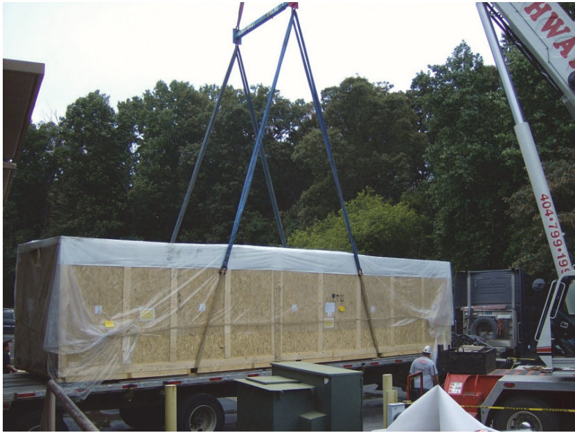
Figure 1-19 Crane Ready to be Lifted
