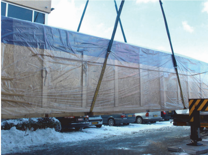
Figure 1-20 Lifting the Crate with the Heavy Crane
