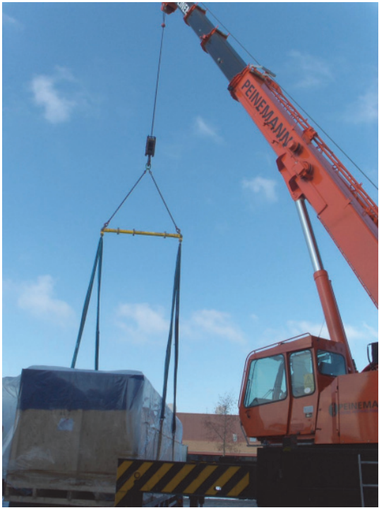
Figure 1-18 Heavy Duty Crane with a Steel Beam and Straps
