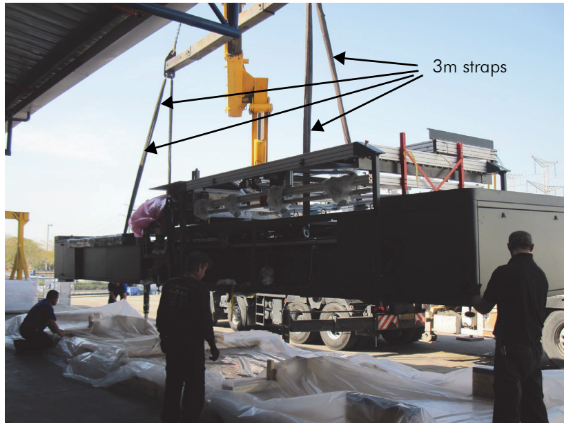
Figure 1-23 Lifting the Unpacked Machine
