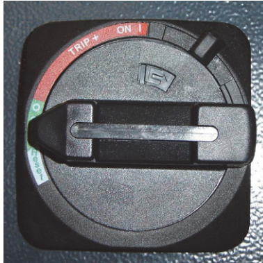
Figure 1-8 UV Main Isolator turned OFF
