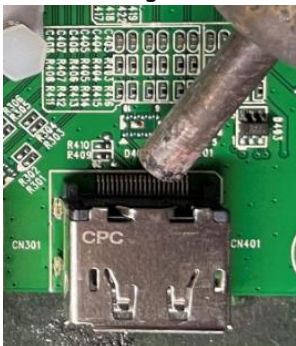
DP connector repairing
